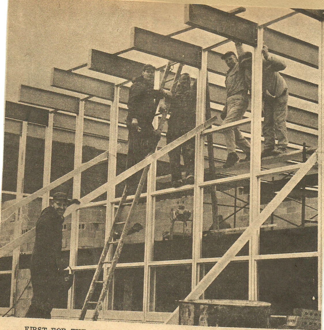
FIRST FOR THE AREA. Something new in construction for this area is displayed as parochial school wing takes shape at Concordia Lutheran church. It is all-aluminum framing. Volunteers on the job above include Grant Warren, 243 East Wilson; Al Titts-worth, 7904 Mildred; Art Hyland, R. R. 4; Willy Hohlick, Chicago; Bob Warren, 243 East Wilson.
